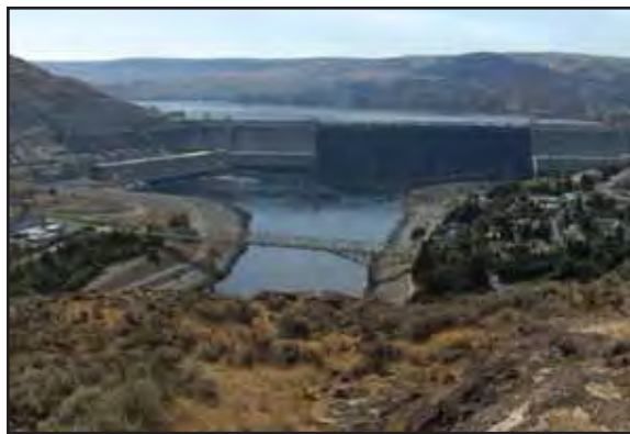
Grand Coulee Dam, Washington
