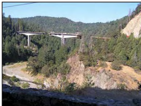
The requisite "bridge under construction" shot.
